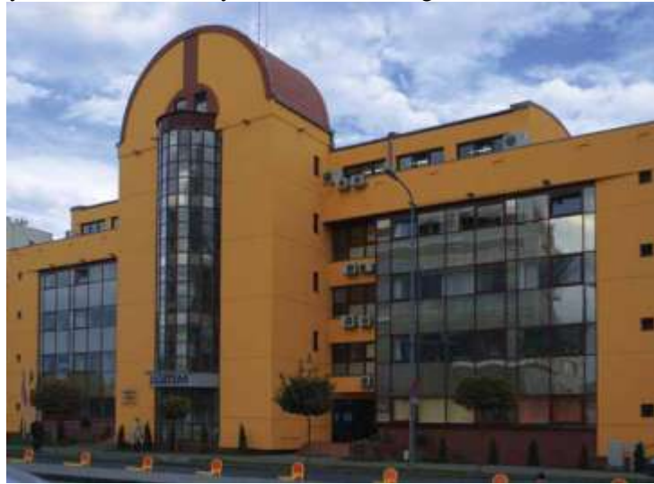
Figure 2. - SC AQUATIM SA building office.
